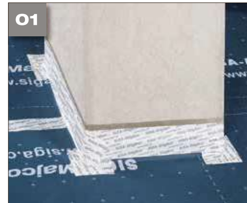
Example at a chimney:
