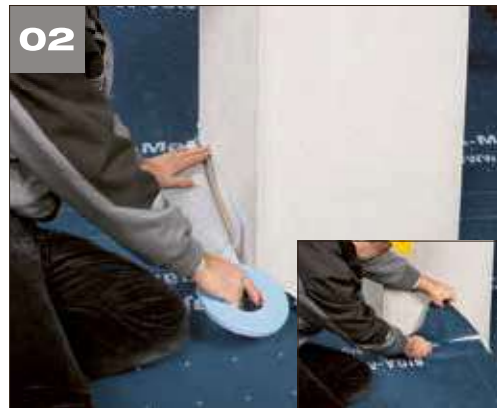
Example at a chimney:
