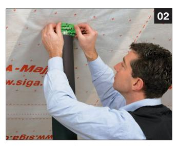
Apply Rissan half to the pipe and half to the the vapour control layer without tension
